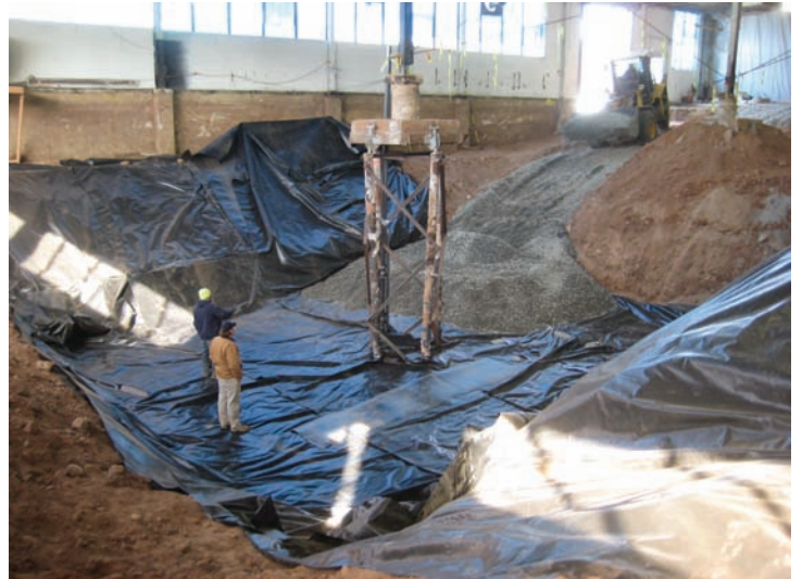
Installation of multi-level vapor barrier system 18 feet beneath building floor slab
