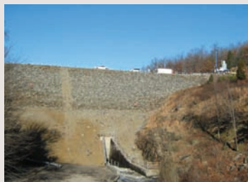
Preliminary testing for grout curtain in earthen dam
